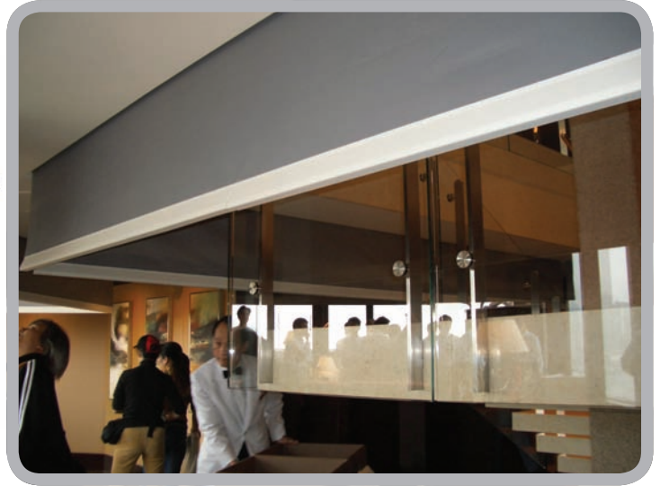
Intercontinental Hotel, Hong Kong - Abutting Single Rollers with minimised edge gap
